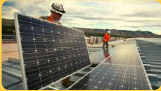
Solar Cell 2 MVA
