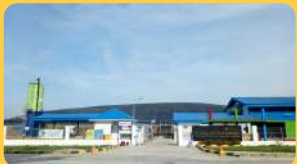
Bio-Gas Power Plant 10 MVA
