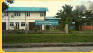
Bio-Mass Power Plant 15 MVA
