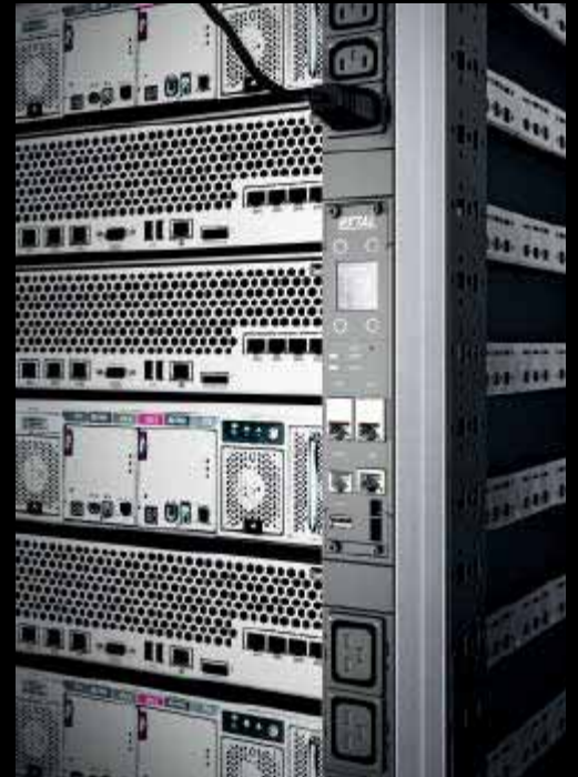
PDU – Socket strip in a rack
