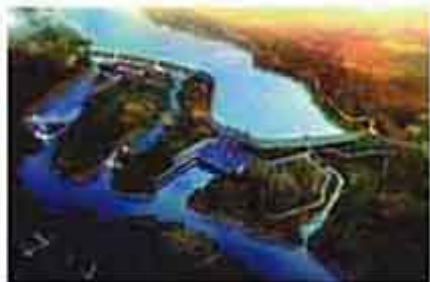
Keleta Hydropower Station, Guinea
