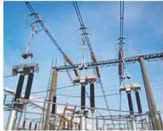
Pantograph Disconnector (126kV-550kV)
