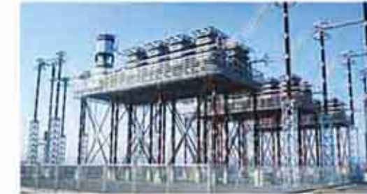
The Jindongnan-Nanyang-Jingmen UHV AC transmission project 1000kV Changzhi Substation, Series Compensation capacity: 1503 MVAR Client: State Grid Corporation of China
