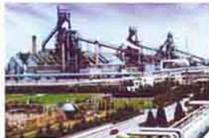
Zhongpu Steel Iron Co., Ltd. 110kV Substation
