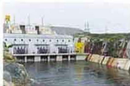
Cote d'Ivoire Subley Hydroelectric Power Station
