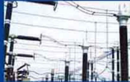
LVB-550 Oil Immersed Inverting Current Transformer Running in Zhejiang Electric Power Company
