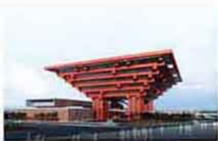
Shanghai World Expo 220kV Mengzi Station
