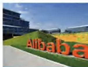
Alibaba Ding computer room project
