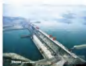
Yichang Three Gorges Dam Project
