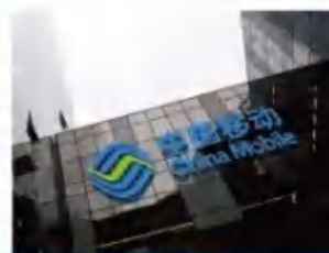
China Mobile Shanghai Jiaxing project
