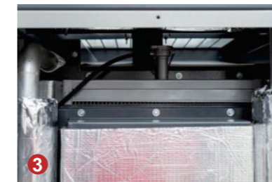
3 Residential level muffler significantly reduced the engine noise.
