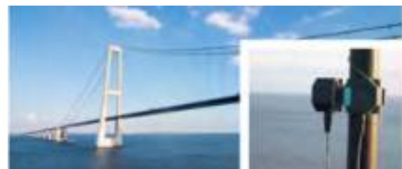
Figure 4.17 Accelerometer attached to a bridge's structure (Source: © 2024 Kistler Group/Shutterstock.com)
